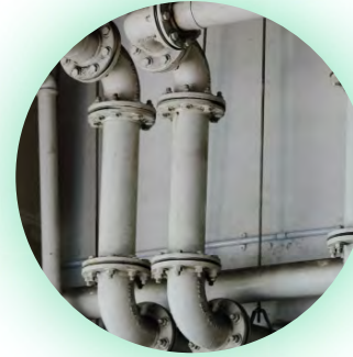
PLUMBING & FIXTURE UPGRADES
